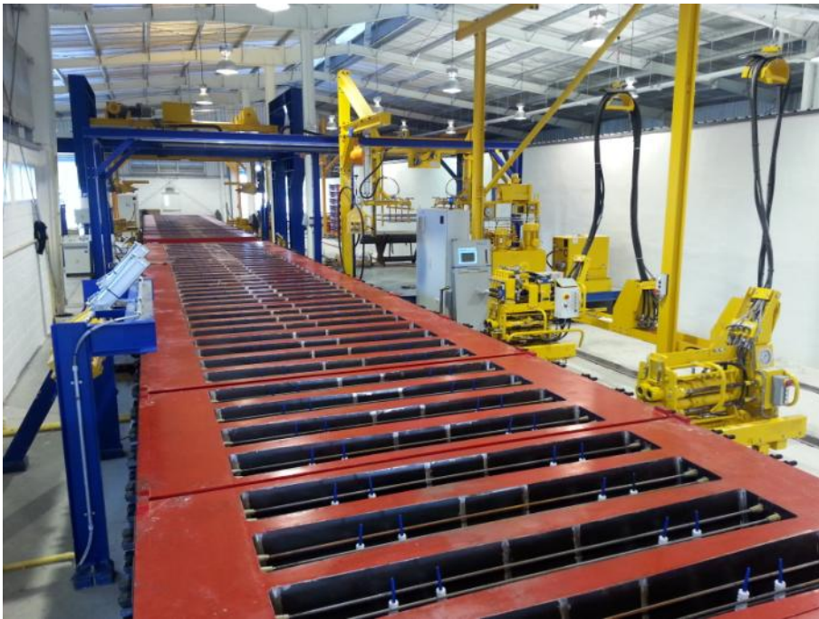
Fig. 4: The prestressing steels are semi-automatically prestressed with a tensioning force of 460 kN.
