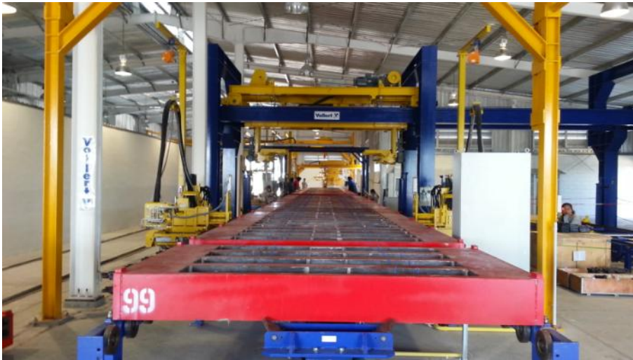
Fig. 9: The prestress release process is subsequently initiated via a semi-automated detensioning station.
