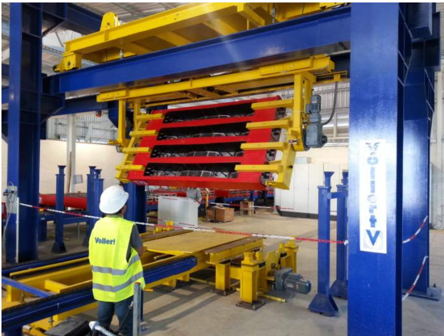
Fig. 10: A turnover spreader beam moves the detensioned concrete mould into an exit area and rotates it by 180 degrees before the demoulding process is performed by an electric lifting mechanism.
