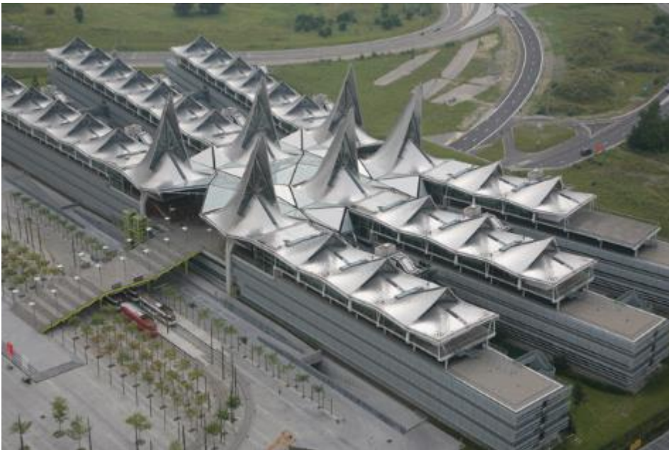
Image 1 + 2 (Source: Kerkstoel 2000+) Modern architecture with precast concrete elements from Kerkstoel 2000+.
