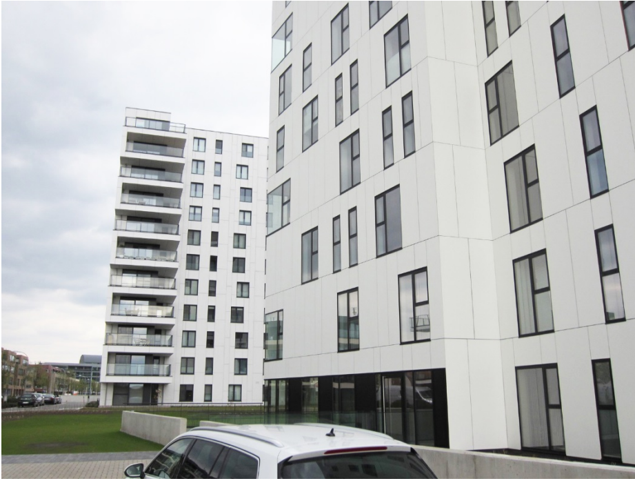
Fig. 9: The modern, attractive architecture is a special characteristic of all projects of the Cordeel Group
