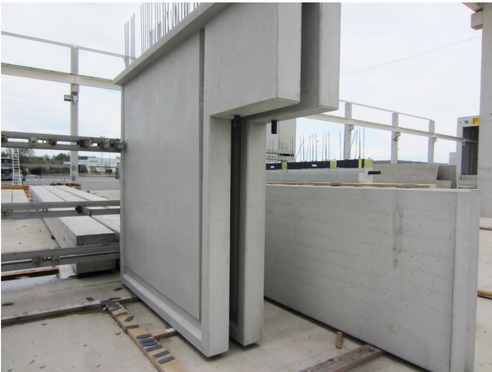
Fig. 8: For the modern architecture in precast concrete construction Cordeel uses solid, double and sandwich concrete parts
