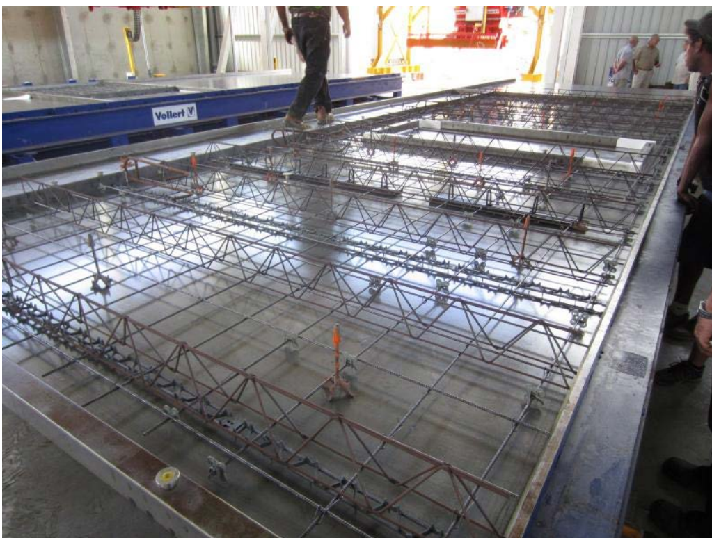
Fig. 4: Reinforcing, concreting and compacting with state-of-the-art plant equipment
