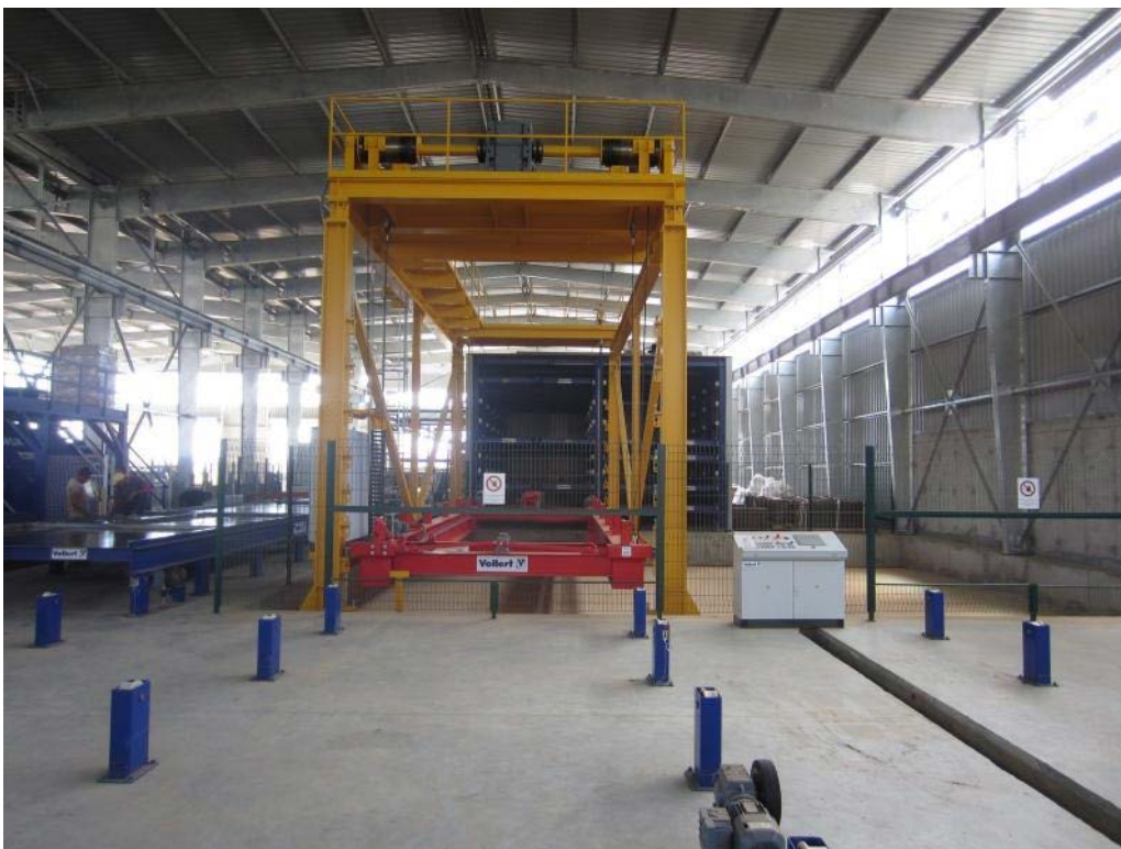
Fig. 6: A floor-guided storage and retrieval machine, which is designed for a pallet area load of 400 kg/m 2 , puts the pallets into storage and removes them again fully automatically
