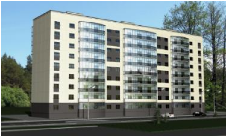
Fig. 8: TOO Bolashak relies on state-of-the-art technology with the construction system for multistorey residential and industrial buildings developed by Elticon
